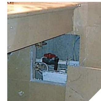
Sanipack installed behind the wall with an access cover
