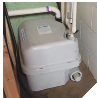
Sanicubic 2 duplex grinder system
