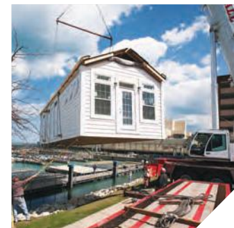
Crane used to place the bathhouse onto the floats
