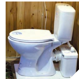
WC installation in the «Bannya» with a Saniflo unit
