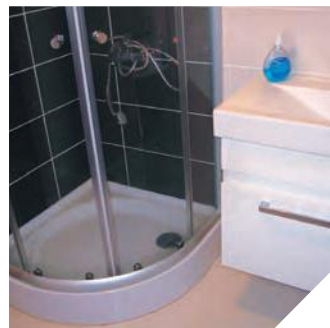
Shower connected to Sanishower concealed behind the wall
