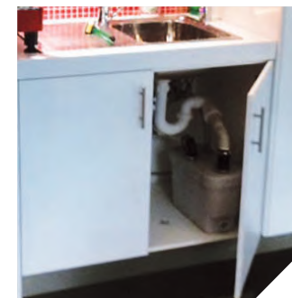
Sanispeed concealed in a sink cabinet
