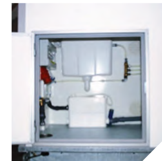
SFA unit recessed behind an access door handles the waste
