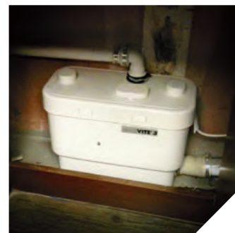
Sanivite concealed in a sink cabinet
